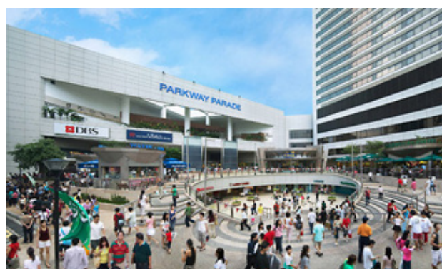
Lend Lease’s Parkway Parade – One of the first BCA Green Mark Platinum certified retail and office buildings in Singapore
