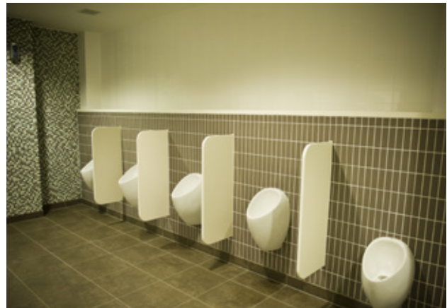
Top: Stockland’s Northshore Mall in Queensland Above: Many Stockland Malls feature waterless urinals
