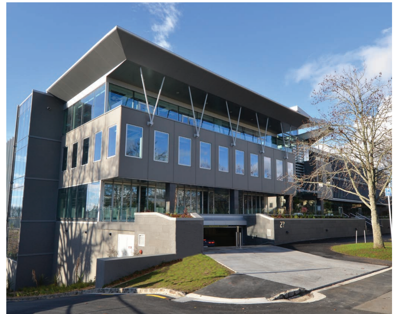
The GHD Building in Freemans Bay... one of a number of Green Star rated buildings developed by Mansons TCLM.
