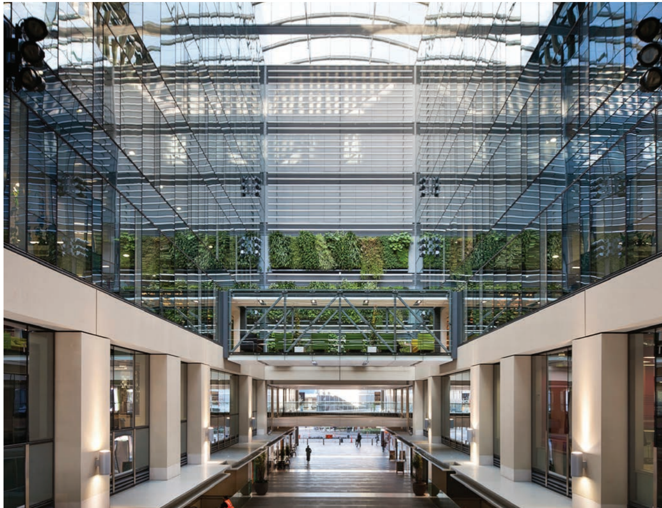
The green wall... the 5 Green Star Westpac on Takutai Square Building in Auckland's Britomart precinct.
