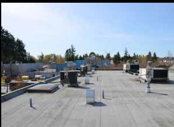
View Of Recently Replaced "Torched on" Roof
