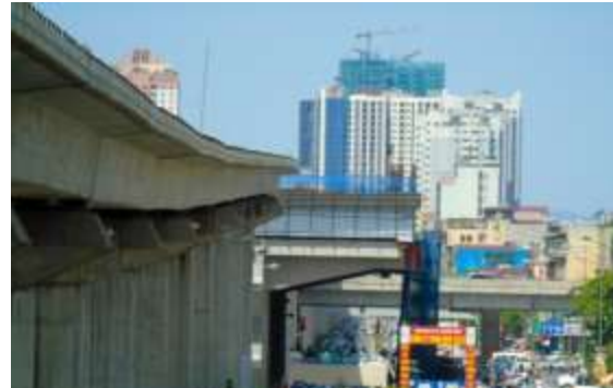
Depot on Nguyen Trai Road & Ring Road No.3
