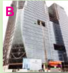
B HUD TOWER Cau Giay Dist. 56,000 sqm
