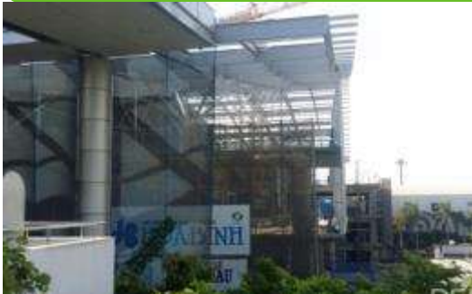
HCMC – airport expansion under construction
