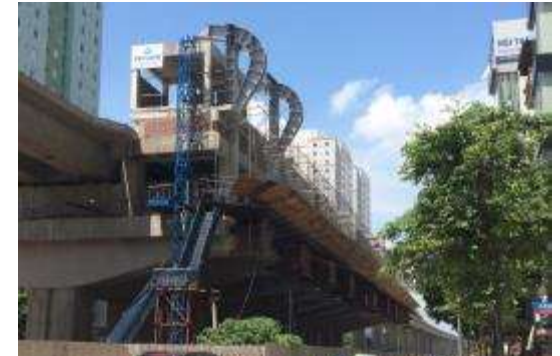
Depot on Nguyen Trai Road, Ho Guom Plaza
