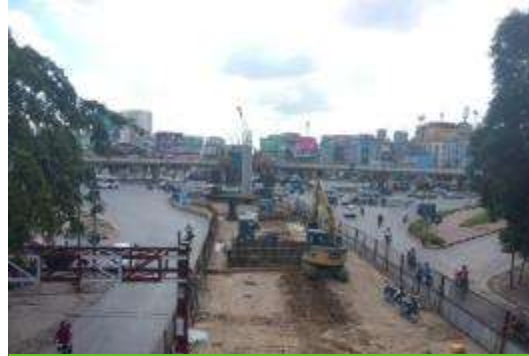
Depot on Cau Giay – Pham Hung Intersection
