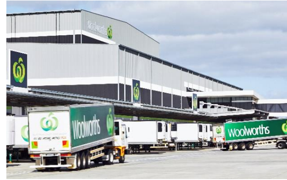
Woolworths Distribution Centre, Dandenong, Melbourne
