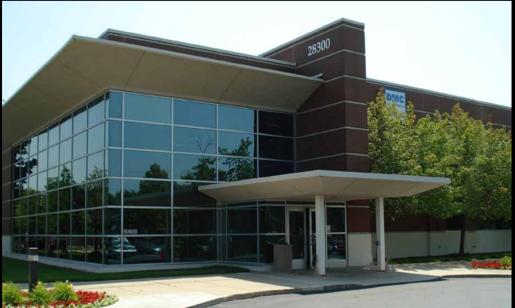
DMC Medical Office Building 28300 Orchard Lake Road | Farmington Hills, MI
