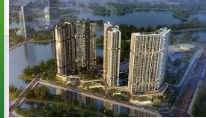
Project at Gamuda City ~2,000 units
