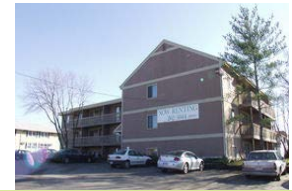
EAST VILLAGE PARK APARTMENTS
