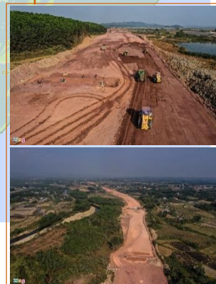
Construction of Van Don - Mong Cai Expressway is expected to complete in 2021.
