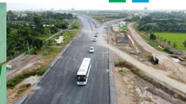
Experimental operation of Trung Luong - My Thuan Expressway in December 2020.
