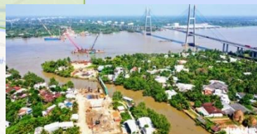
Construction of My Thuan 2 Bridge started in August 2020.
