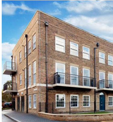
Brick returns along the side
