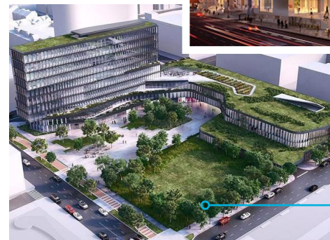
CUMMINS INC. FUTURE DISTRIBUTION HQ One city block bordered by Market, Alabama, Washington & New Jersey Streets
