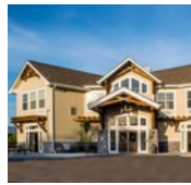
Cappella of Grand Junction Confidential Grand Junction, CO 66 AL/MC units Client was Confluent Senior Living
