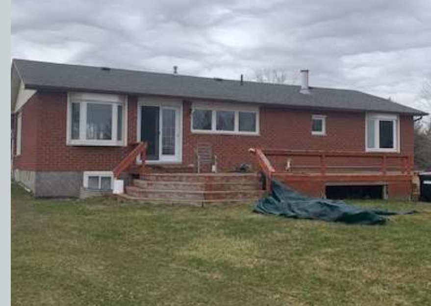
Rear of House
