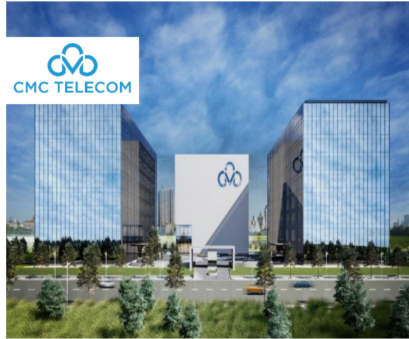
CMC Space – Tan Thuan Industrial Park – D.7, HCMC Land Area: >13,000 sqm Under construction
