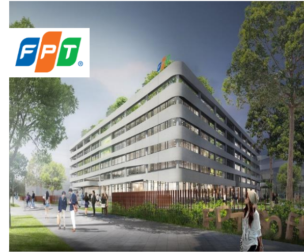
FPT R&D Center – Hi-tech Park Long Thanh My Ward, D.9 Land Area: >42,000 sqm Under construction
