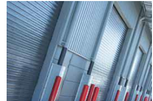
Willawong Logistics Facility 237 Gooderham Rd, Willawong QLD
