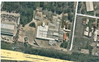
Huntingwood East Logistics Park Flushcombe Rd, Huntingwood NSW
