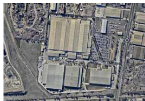
Fitzgerald Rd Distribution Centre 63-83 Fitzgerald Rr, Laverton VIC
