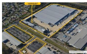
Minchinbury Dist. Centre 1 Sargents Rd, Minchinbury NSW
