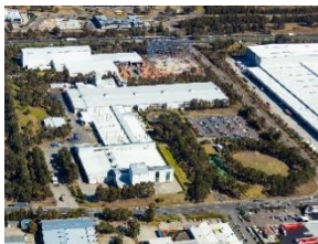
Huntingwood Distribution Facility 61 Huntingwood Dr, H'wood NSW
