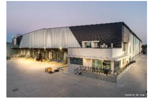
Chullora Logistics Park 2 Hume Highway, Chullora NSW
