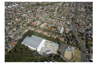
Greenacre Logistics Facility 1 Moondo St, Greenacre NSW
