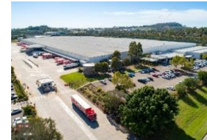
Smeaton Grange Dist. Centre 80 Hartley Rd, Smeaton Grange NSW
