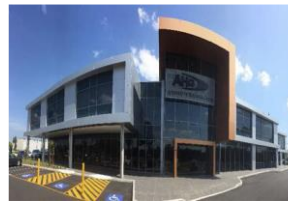
Prestons Distribution Facility 402 Hoxton Pk, Prestons NSW
