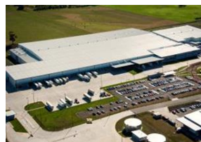
Translink Distribution Centre 4-20 Translink Ave, Launceston TAS
