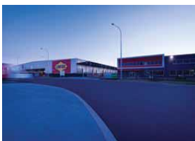
Stockyards Industrial Estate 385 Bushmead Rd, Hazelmere WA
